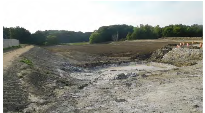
This photo looks west behind the Deer Wood Estates subdivision, north of Lakeshore Blvd.
